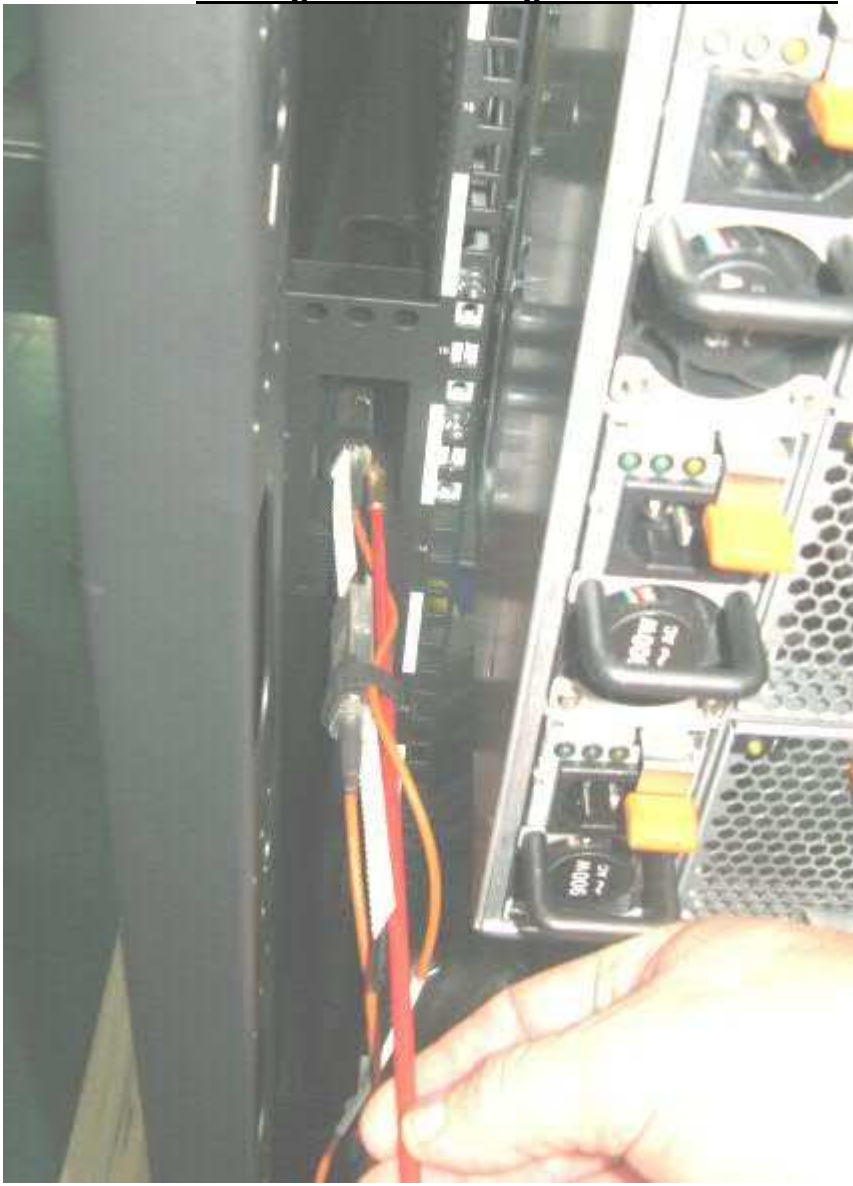
Fishing Cables Through Cable Channel #3
