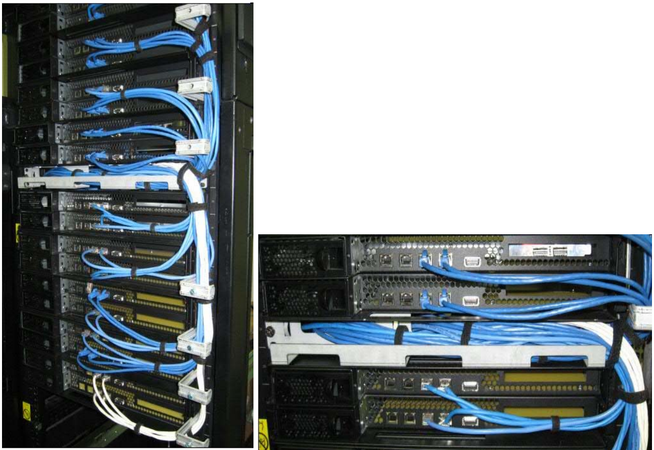
Rack cabling with 1U cable management bracket.
