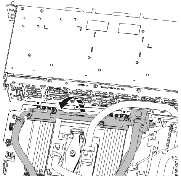
Figure 14. Moving the front pipe away
