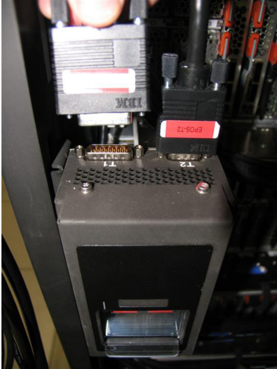
Figure 12 UEPO Cable Removal
