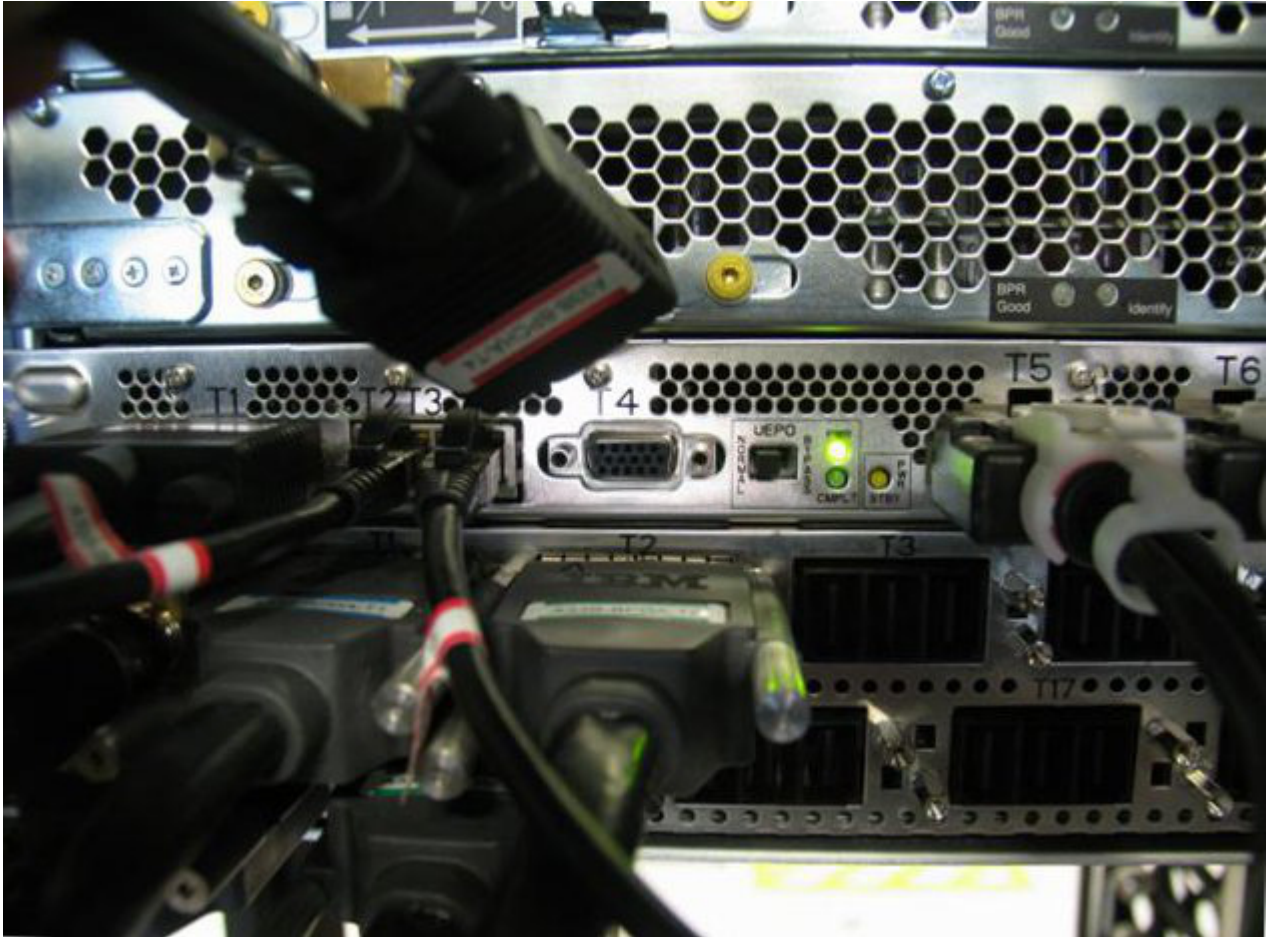
Figure 13 Removal of UEPO Cable from BPCH T4
