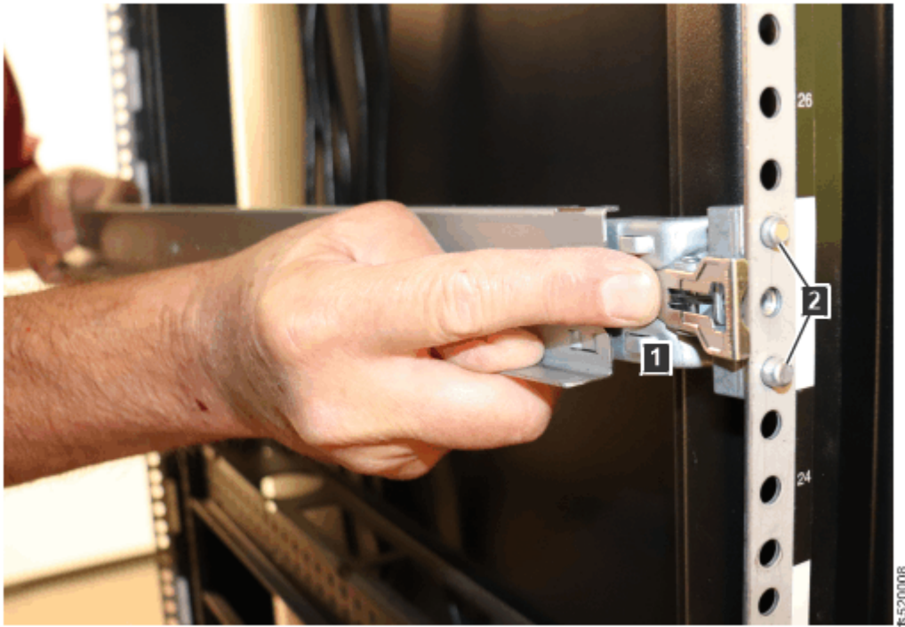
Figure 66. Installing the rear rail bracket
