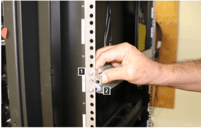
Figure 29. Installing the front rail bracket
