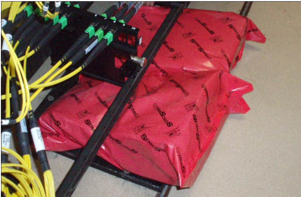
Figure 4-2 Sealed tile with pillows
