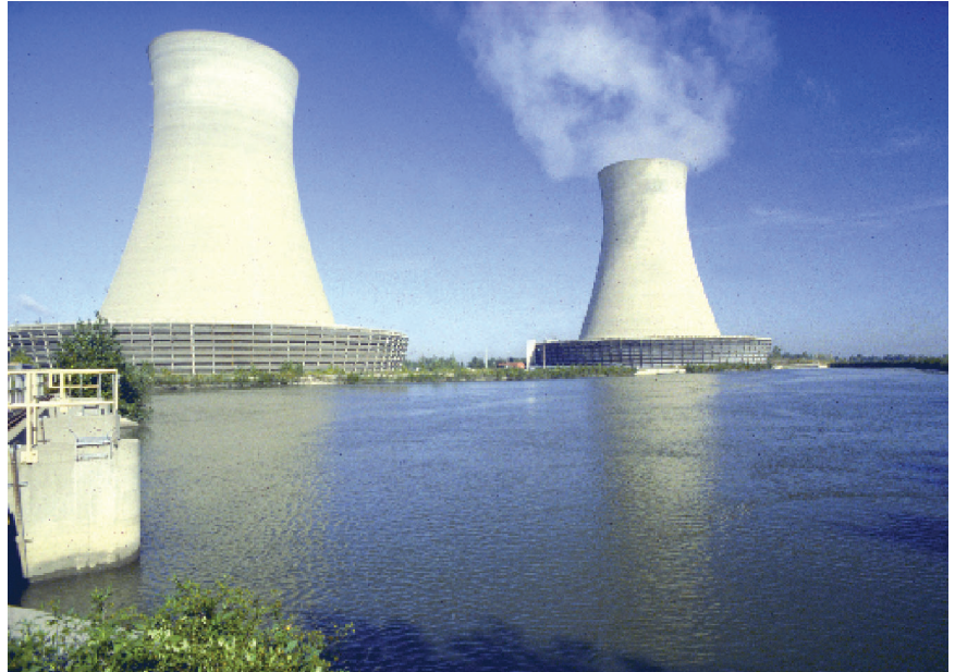
DTE Energy is a 150-year-old company with $9B in revenues and manages $23B in assets. These include Detroit Edison with 2.2 million electric customers, nine fossil units, and the Fermi 2 nuclear power station, generating 11,000 megawatts, as well as MichCon, serving 1.3 million gas customers in Michigan. DTE Energy operates non-regulated businesses in 38 states.
