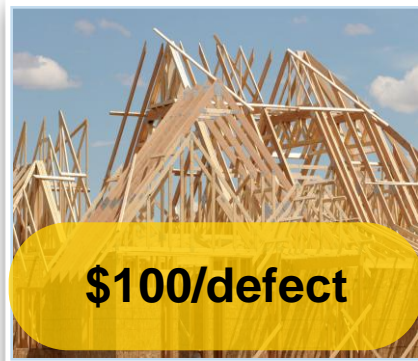
During the build phase
