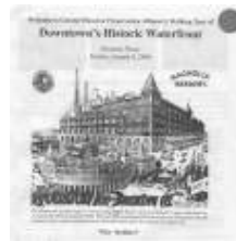
The Louisiana Ice Manufacturing Company Automated Manufacture
