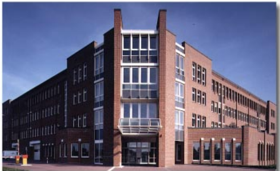
GAD Data Centre, Muenster, Germany
