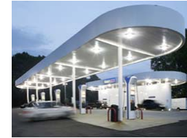
Caisse automatique Station service
