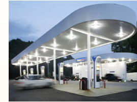
Caisse automatique Station service
