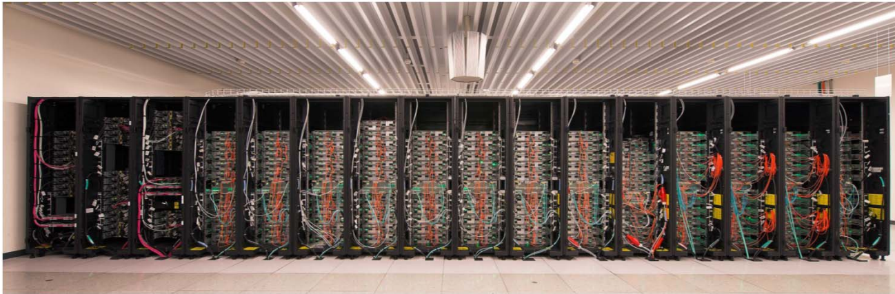
this picture shows 16 of 23 Storage-Racks ( IBM Enterprise Storage ) per location
